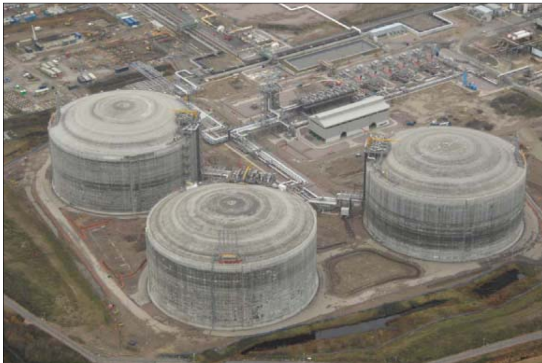
UK's National Grid Grain LNG terminal at yearend 2008 started up an expansion that increased its import capacity by 50%, to 14.8 million tonnes from 9.8 million tonnes. The £310 million investment is supported by long-term contracts with E.On, Iberdrola, and Centrica, which took all the additional capacity. This third phase expansion brings National Grid's investment at the site, according to the company, to more than £750 million and enables the terminal to import around 20% of forecast UK gas demand by 2010-11. (Photograph from National Grid Grain LNG)
