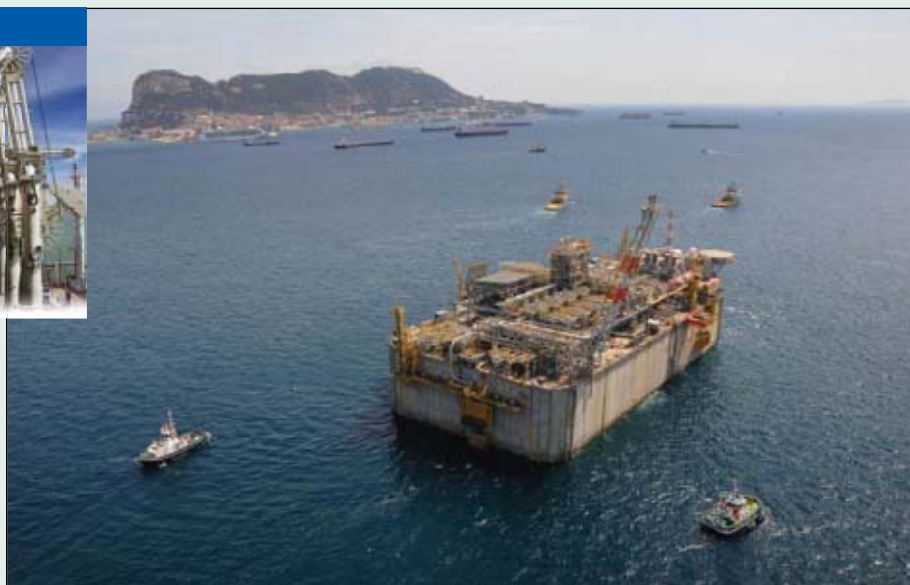
Tugs and tenders near Algeciras, Spain, maneuver the world's first fixed offshore LNG terminal last year as it moves toward its Adriatic station off Porto Levante, Italy (Fig. 2; photo from ExxonMobil).
